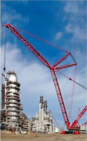
Crawler cranes <300t
