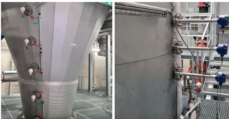
Picture 31: Sensor to check the gasification process.
