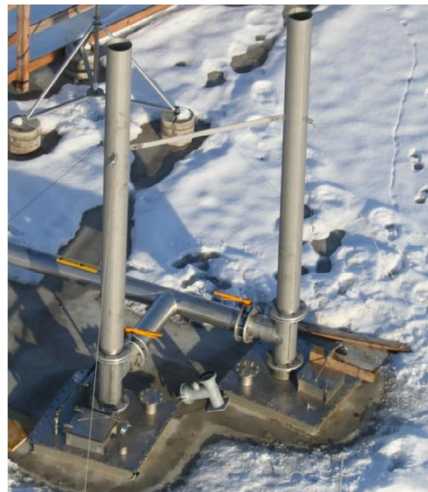
Picture 42: types of over and under pressure valves, Important to notice: no valve has to be installed between valve and digester, exhaust pipe has to be outside of contact area, if installed outside it needs to be secured from freezing.
