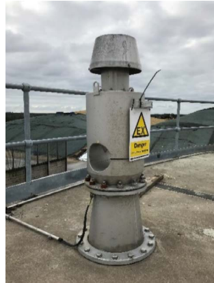
Picture 41: Over and under pressure valve. Important to notice that exhaust pipe must be outside.
