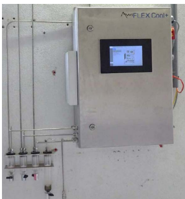
Picture 49: Biogas analysis to detect CH_4 , CO_2 , H_2S and H .
