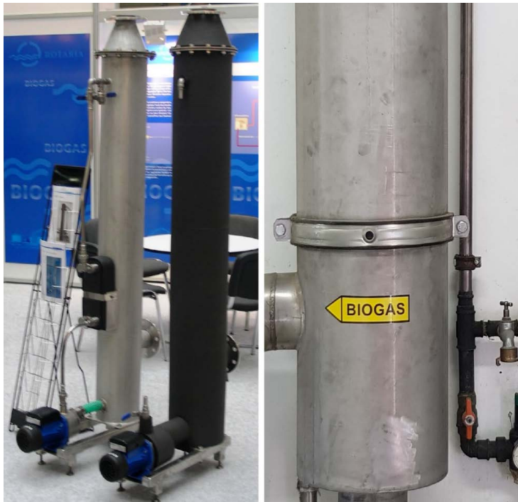
Picture 67: External biogas coolers with integrated particle separator.
