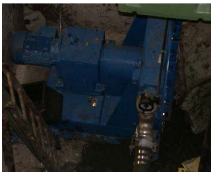
Picture 36: Peristaltic pump.
