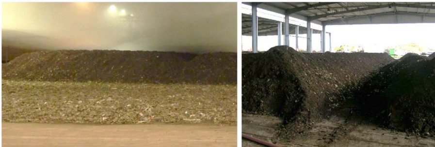
Picture 53: Post-composting of digester from a dry fermentation process; left: in a closed hall with automatic aeration through the compost windrow and collection and cleaning of exhaust air in a biofilter, right: windrow post-composting in an open hall.
