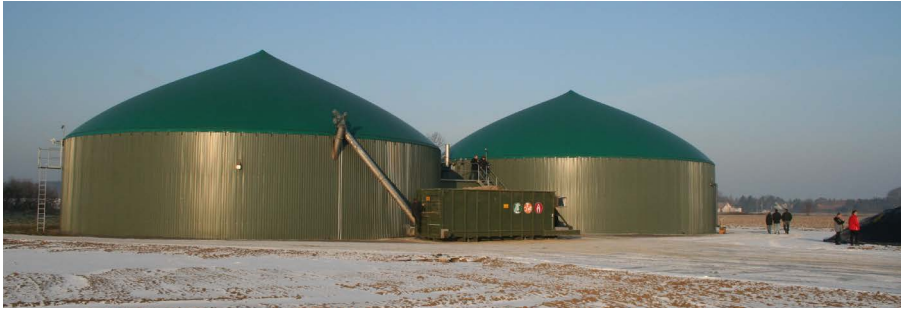
Picture 21: Typical biogas plant with a main digester followed by a post digester.
