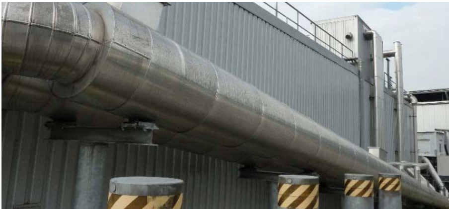
Picture 31: External heat exchanger where the substrate that will be fed gets heated and pressed into the digester.
