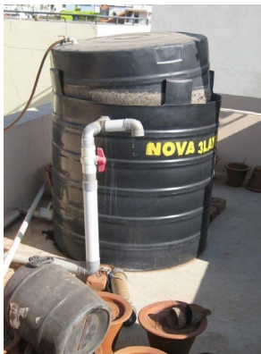
Picture 72: Floating drum digester. Source: German Biogas Association.
