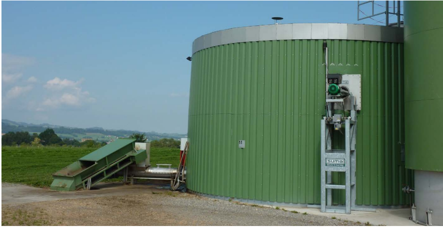
Picture 19: Hydrolysis tank upfront of the digester.
