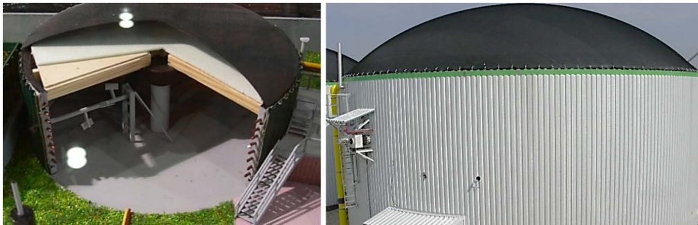
Picture 58: left: cross section of a model with single membrane; right: digester with single EPDM membrane.
