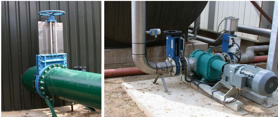
Picture 37: Rotary displacement pump with manually steered (left) and automatically steered (right) valve(s).
