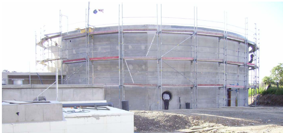
Picture 22: Concrete digester.
