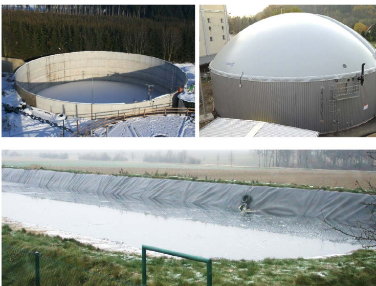
Picture 55: Digestate storage tank: top left: open storage tank, top right: airtight gas storage tank with a double membrane layer and connection to the gas system, below: open lagoon with double layer membrane to monitor tightness.
