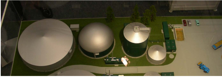
Picture 20: Model of a biogas plant with multistage digestion process (feeder, storage tank for slurry, main digester, post digester, gas-tight storage tank).
