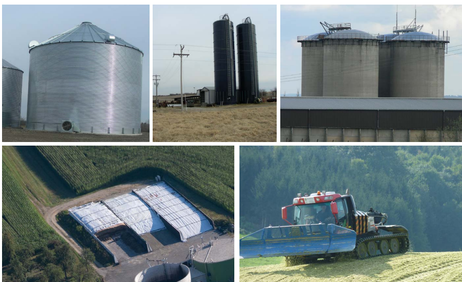
Picture 2: Different types of storage systems: top left: not gas-tight silo, top middle: gas-tight silo where conservation is done with carbon dioxide, top right: air-tight silo where conservation is done through lowering pH value, bottom: air-tight clamp silo, where compression is done with heavy machinery like tractors or even snow groomers.
