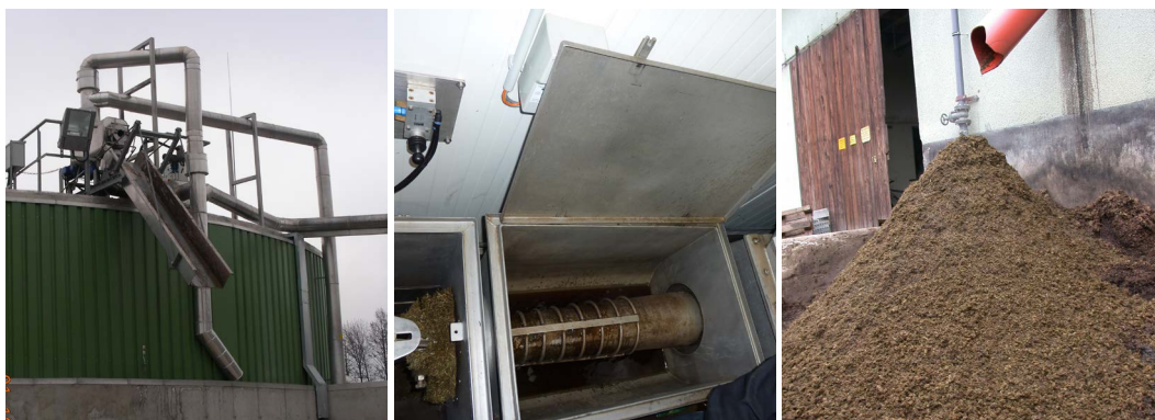
Picture 38: Rotary piston pump with rubber puffer on both sides to avoid vibration damage and pressure measurement devices before and after to detect vacuum or too high pressure.
