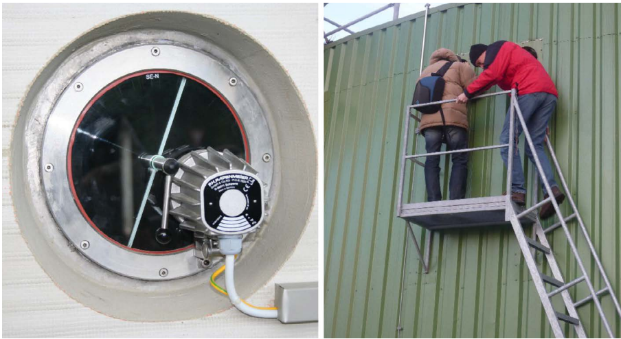
Figure 21: left: inspection hole with camera system, right: manual inspection.
